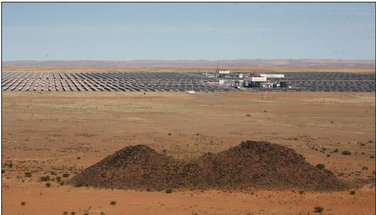
Figure 26. Looking south from the hills along the road to Onseepkans over the CSP plant that is located east of the Paulputs substation. Existing impact in the area consists of the two CSP plants side by side at site and the Konkoonsies 10MW and the under construction 75MW PV plant south of the Paulputs substation.
