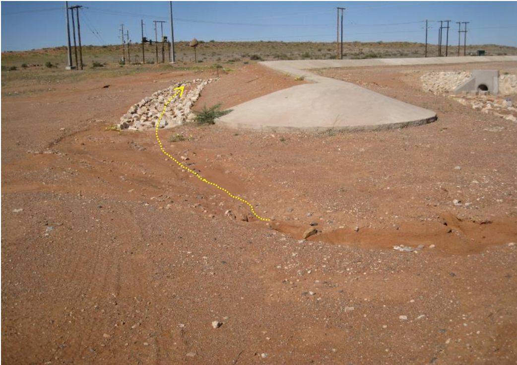
Figure 11: Channel carrying surface water around the Eskom substation (yellow arrow).
