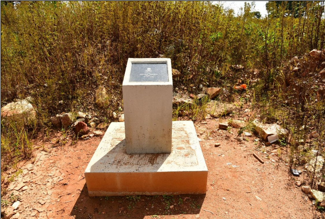
Figure 17: DMR Closed Vertical Mine Shaft (CMR-R66 Vertical Shaft 18/10/2016)
