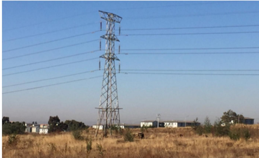
Site Photo 6: View south of the existing power line along which the proposed power line would be routed.
