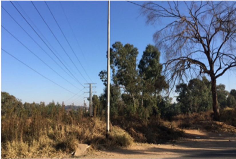
Site Photo 5: View west where the proposed power line routing crosses Hebbard Road alongside the existing power line.
