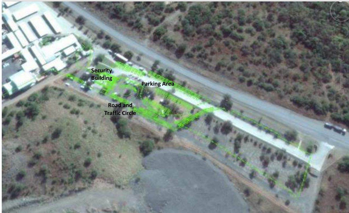
Figure 17: Security Office Upgrades
