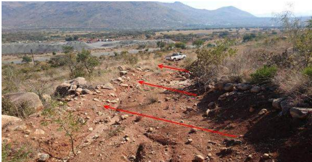
Figure 76: Proposed positioning of berms across an access road
