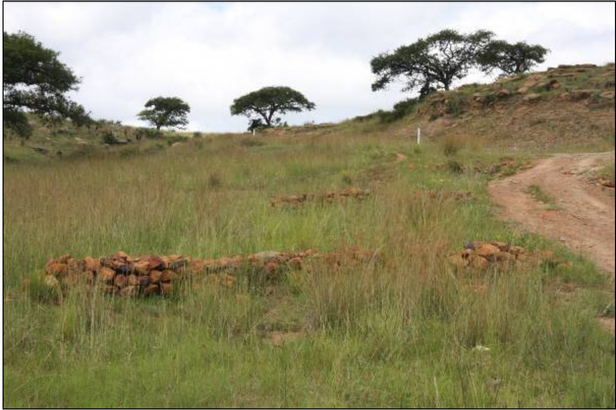
Plate 16. Erosion control measures used to reduce erosion risks on steep slopes
