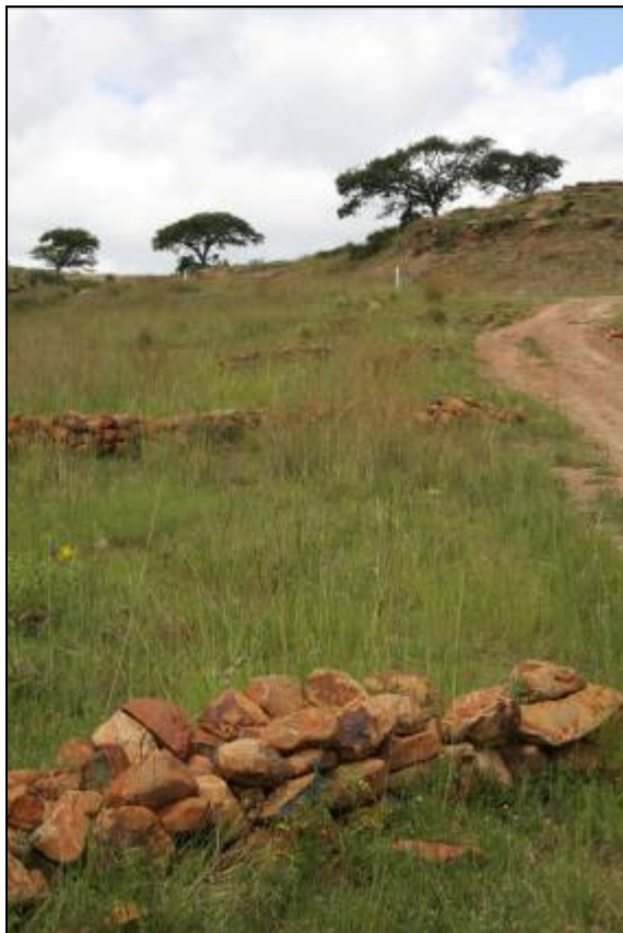
Plate 23. Erosion control measures
