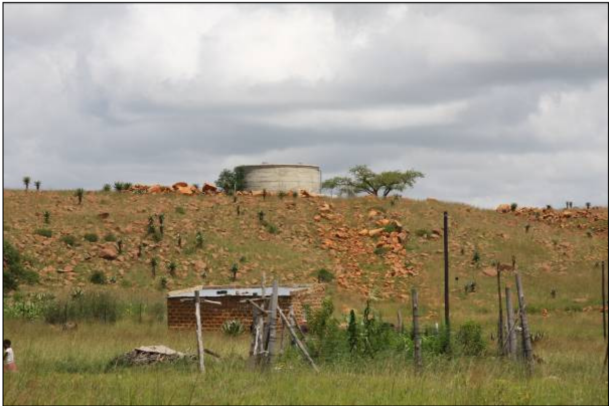
Plate 15. Wasbank Reservoir already constructed and awaiting bulk water supply feed.
