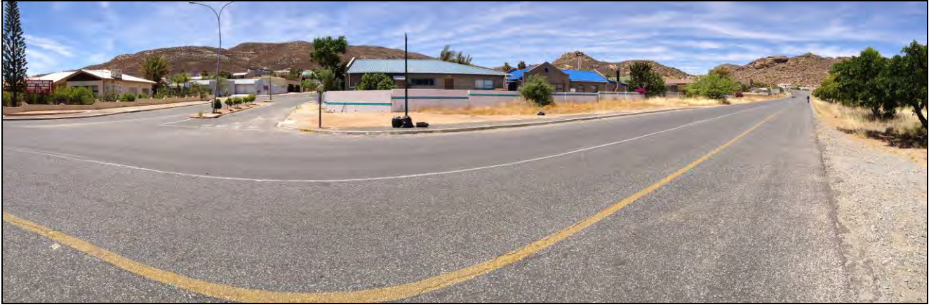
View of Voortrekker street along the site
