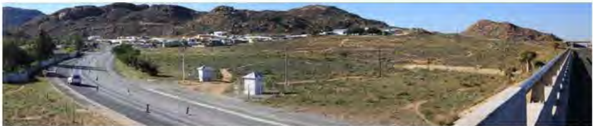
Photo Plate 5 – Proposed site of development on undeveloped land to the south east of Springbok and N7. N14/Voortrekker road runs along lhs of photo.
