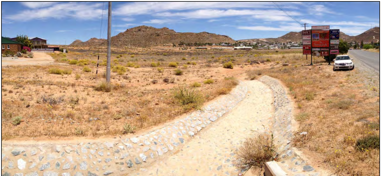
View of the existing storm water channel from neighbouring properties onto the site.
