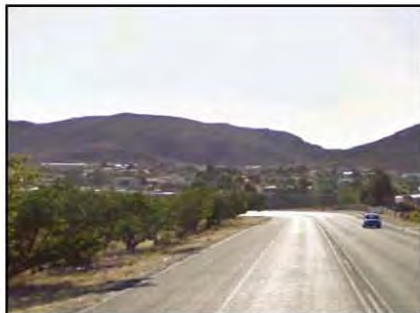
Photo 5: SSD to the west along Voortrekker Street from Main Access
