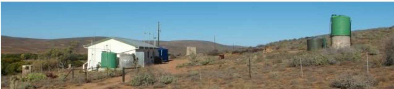
Plate 4.18: Most Project-Affected Farms have water tanks for house drinking water and livestock
