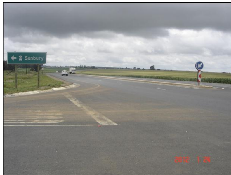
Figure 53: N4 at the Intersection with Sunbury
