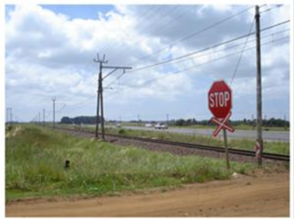
Figure 4: Railway and telecommunication infrastructure.
