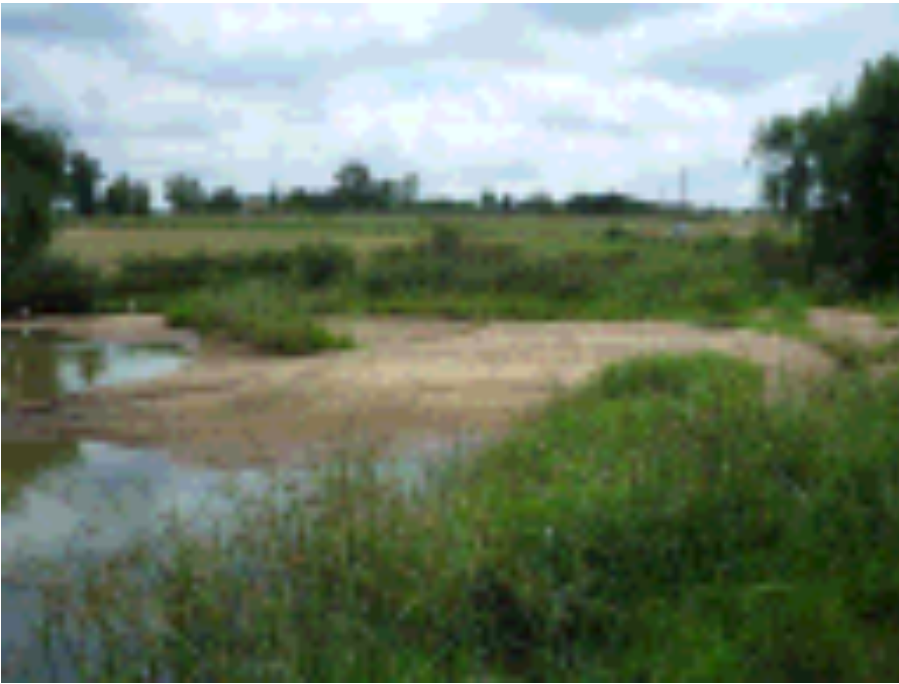
Figure 36 Impoundment with alien vegetation and distinct sedimentation.
