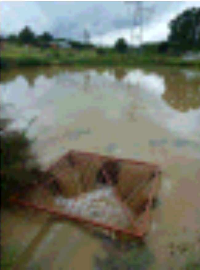
Figure 37 Storm water outflow
