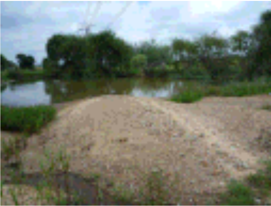
Figure 42 Sediment accumulated in the impoundment.
