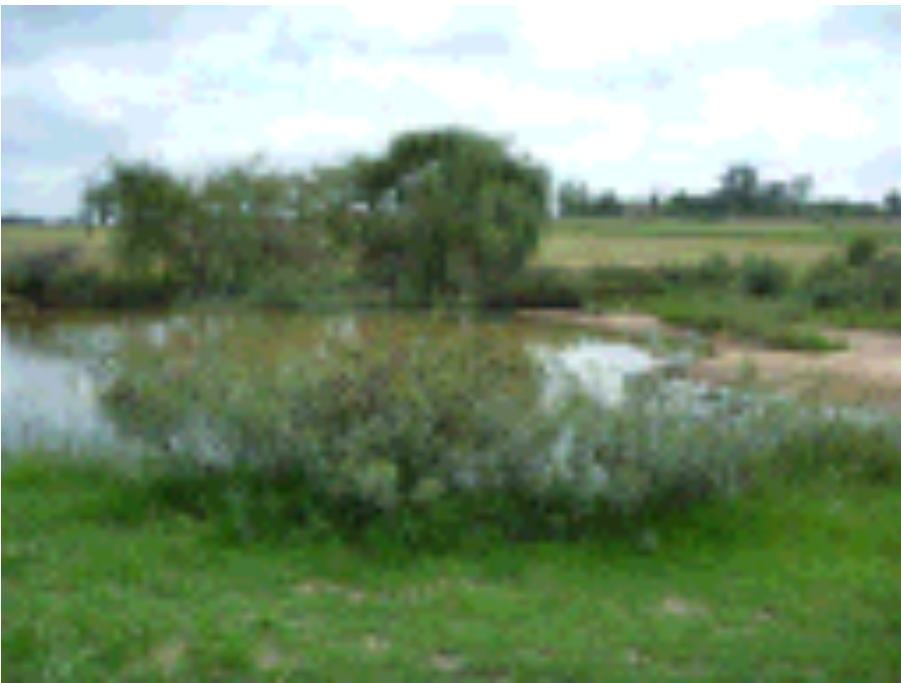
Figure 35 Impoundment with alien vegetation and distinct sedimentation.
