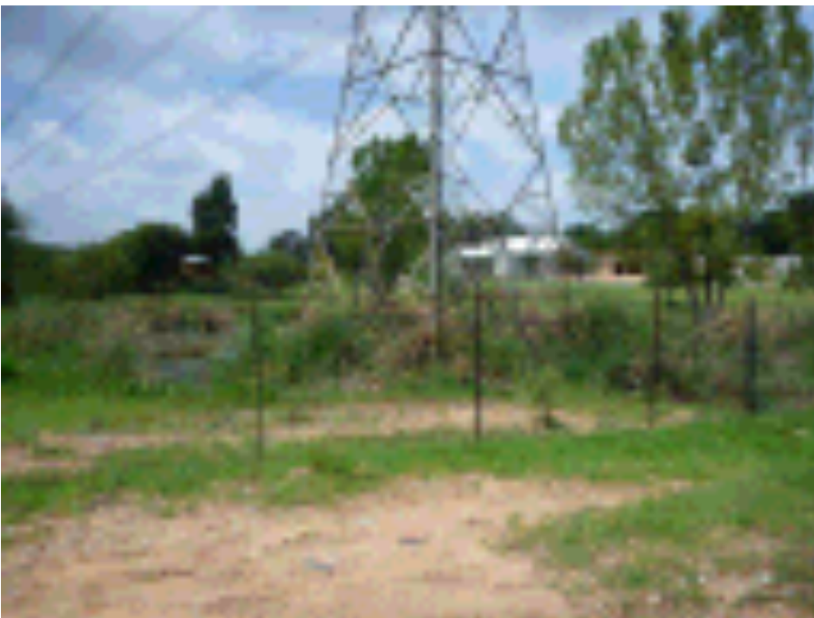
Figure 45 Eskom pylon within the wetland/drainage channel with sediment in the foreground.
