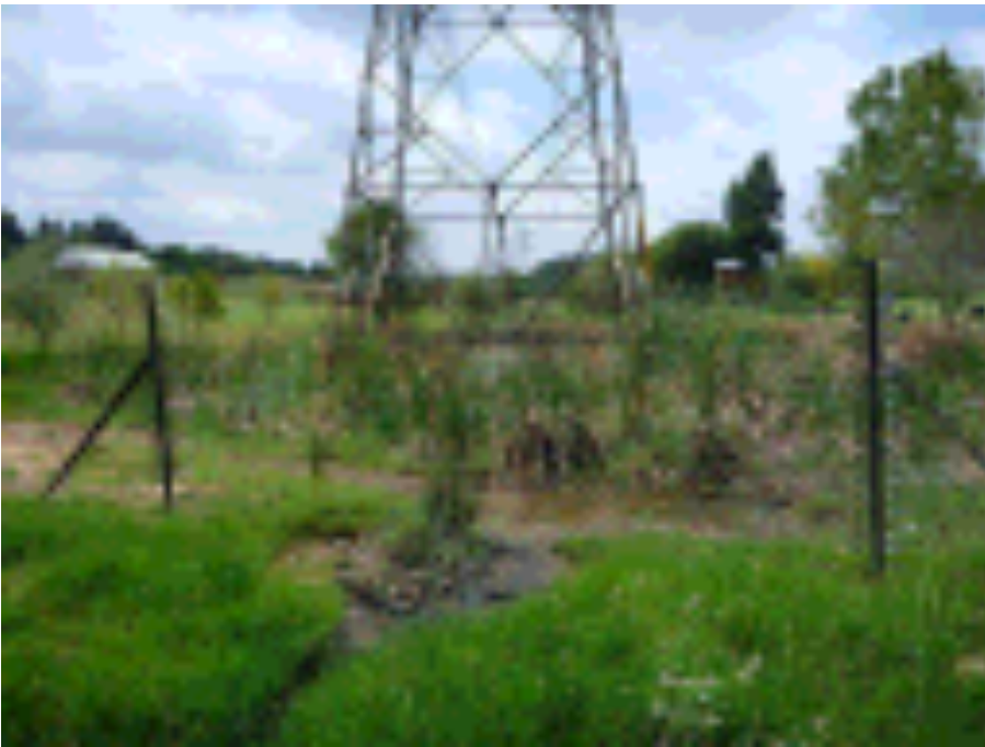
Figure 44 Eskom pylon within the wetland/drainage channel.
