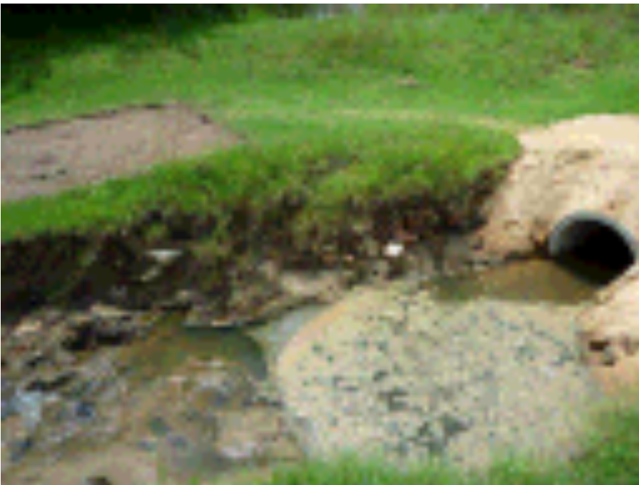
Figure 31 Eroded channel with bricks and rubble visible in the exposed profile indicating historical impacts.
