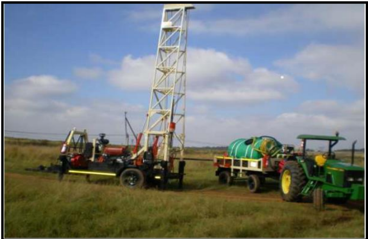
Figure 1-3: Typical LY44 Geological core drill unit
