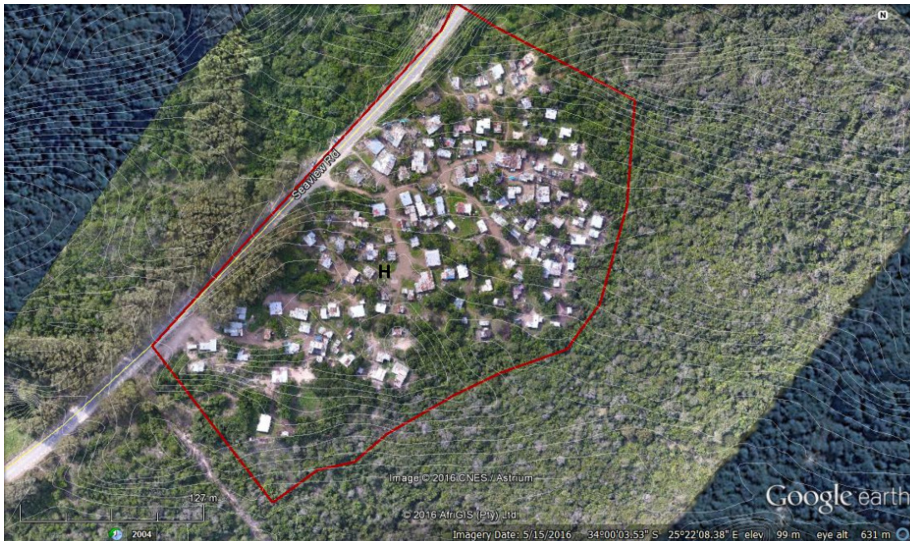
Figure 13: Current and high resolution aerial image of Area H (images provided by Robertson Baker Lochner Architects, 2016).
