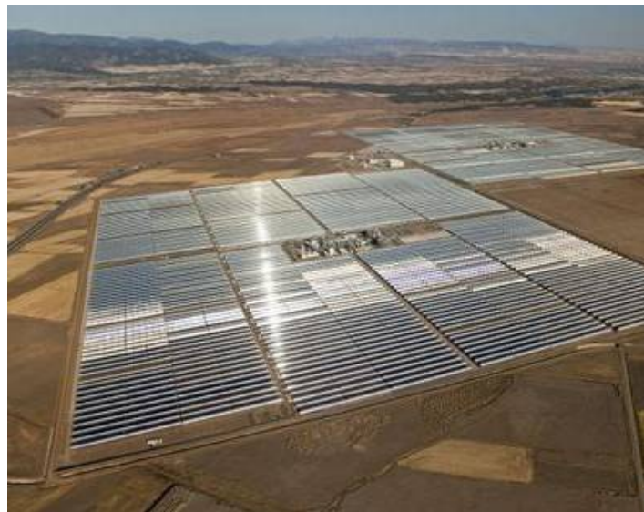
Figure 9: Photographic illustration of the Andasol plant in Spain 8
