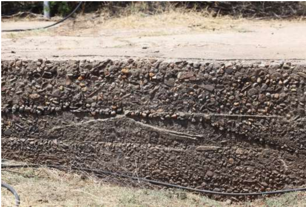
Photo 6 Low concrete wall where road crosses at the northeastern parts of the site, resulting in impoundment of water near an inlet of the Wentzel Dam. Photo: R.F. Terblanche
