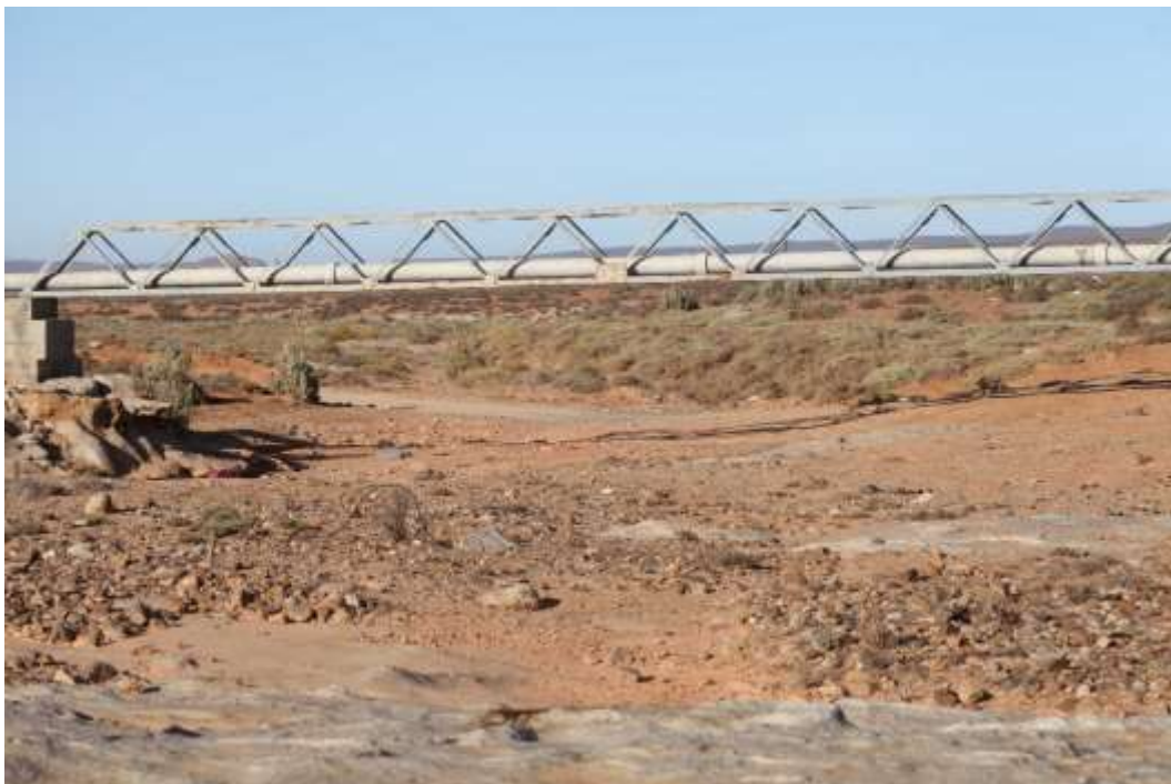
Photo 6 Sewage cross-over at active channel at southwestern part of the site.
