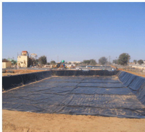
Figure 2.9: A HDPE liner inserted into an excavated pond.
