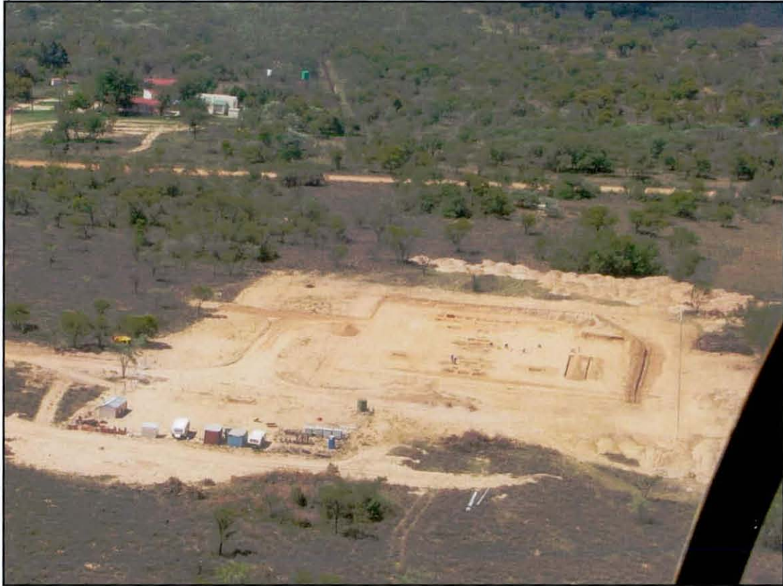
Figure 9. Dorset Substation construction site photographed from a helicopter (Dec.2010)
