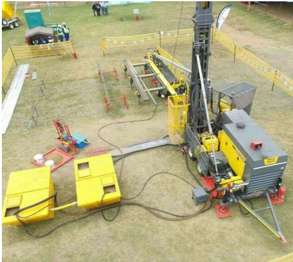
Figure 7: Typical examples of drill rig site
