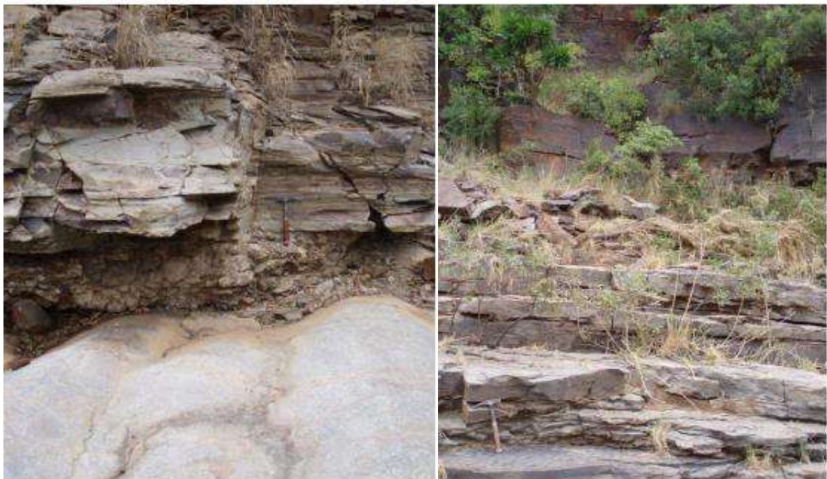
Figure 20: Sharp, locally sheared contact between Klipkloof quartz arenite and Vlakhoek Member shales, Nxobongo stream, Denny Dalton sector. Photo facing northeast
