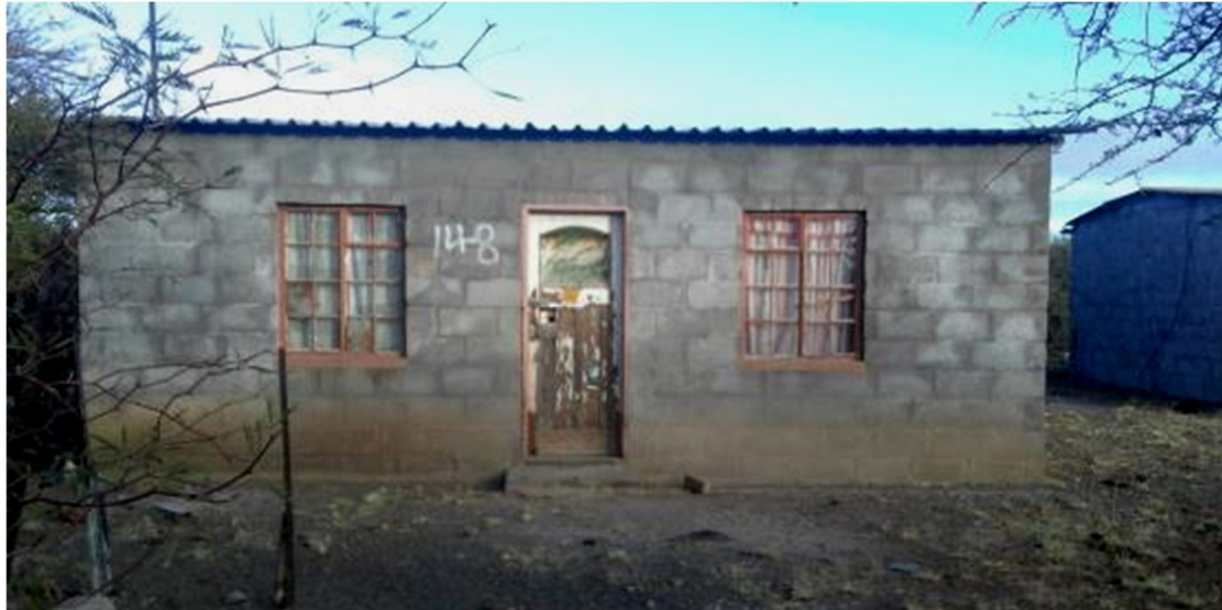
Fig. 25. In the two other labourers quarters buildings we again find the anomaly of an old door and frame possibly dating to the 1930s with modern cement bricks and modern steel frames as part of the building. (Photo S.M. Miller 2018.)
