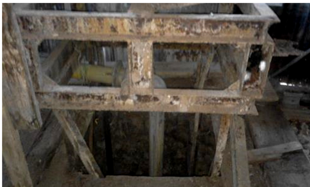
Fig. 37. The original farm well now enclosed in this corrugated iron building. As can be seen water is now being directly pumped from the well for the cattle on the farm. This well is protected under the 60 year rule of act 25 of 1999. (Photo S.M. Miller 2018.)
