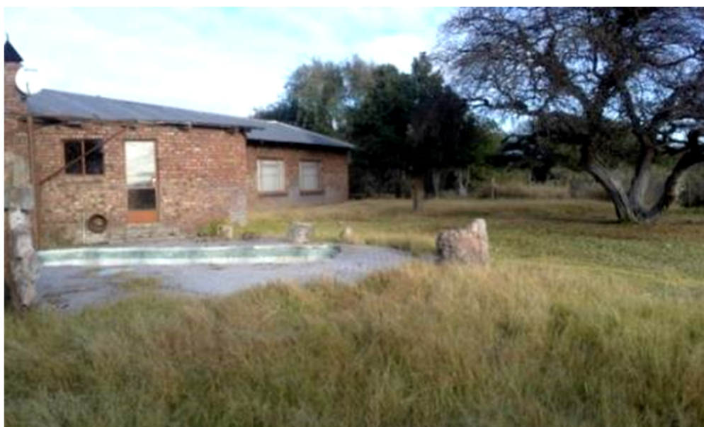
Figs. 10 to 12. Aspects of the present farmhouse that dates to the 1970s or 1980s. This building is not protected by act 25 of 1999. (Photos S.M. Miller 2018.)
