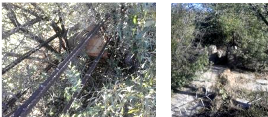
Figs. 53 and 54. This is the remains of a sheep dip that is obviously constructed of modern materials and is not related to the first phase occupation of the farm. This is not a protected structure. (Photos S.M. Miller 2018.)
