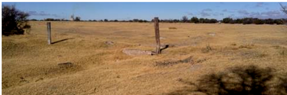
Fig. 46. The sluice gate control from the pans to the irrigation fields on the eastern part of the property. (Photo S.M. Miller 2018.)
