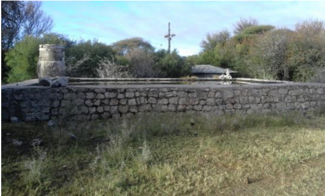
Fig. 30. Northern aspect of the water reservoir. Even though if it is difficult to place the structure beyond the 60 year rule, it is still a remarkable structure associated with farming in the Northern Cape. Local limestone blocks rather than concrete or bricks were used for its construction. The reservoirs position, adjacent to the well and the original water source, points in the direction that it was one of the first structures erected for the management of water resources of the farm in the beginning of the 20 th century. (Photo S.M. Miller 2018.)
