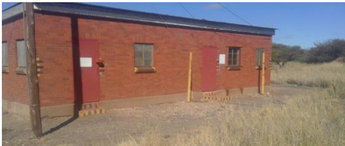
Fig. 64. Ghaap station. This is not a station building but merely a building containing the signal control system for this section of the railway line. (Photo S.M. Miller 2018.)
