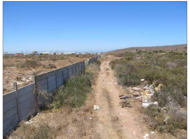
Figure 10. View along vibracrete wall facing south
