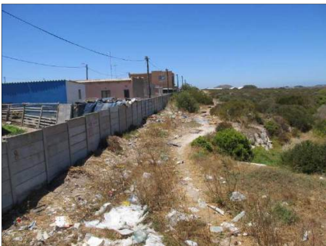
Figure 11. View along vibracrete wall facing east
