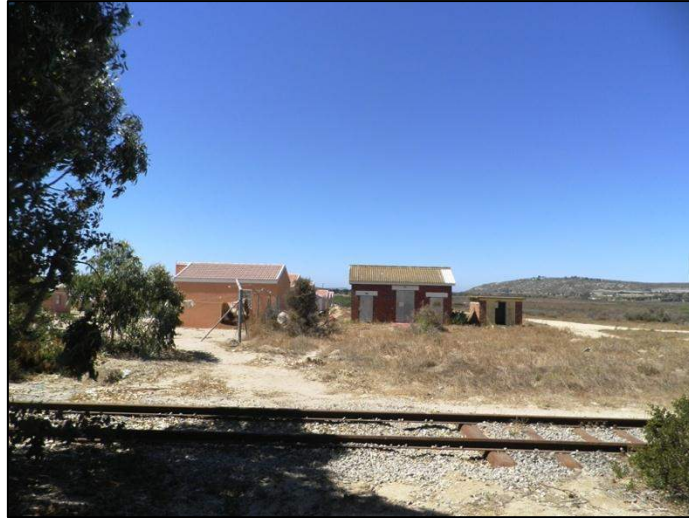
Photograph 2.21: Non-defined housing development on former Saldanha military land. Military structures (right of housing) are an electrical substation and a WW2 bunkers both under threat of constant vandalism from civilians, 2013 O'Donoghue
