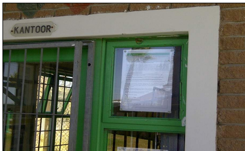
Site Notice 3: Saldanha Post Office
