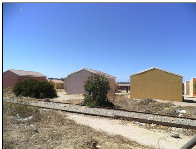
Photograph 2.20: Existing disused military infrastructure (railway line) situated adjacent to RDP housing development on former Saldanha military land, 2013 O'Donoghue
