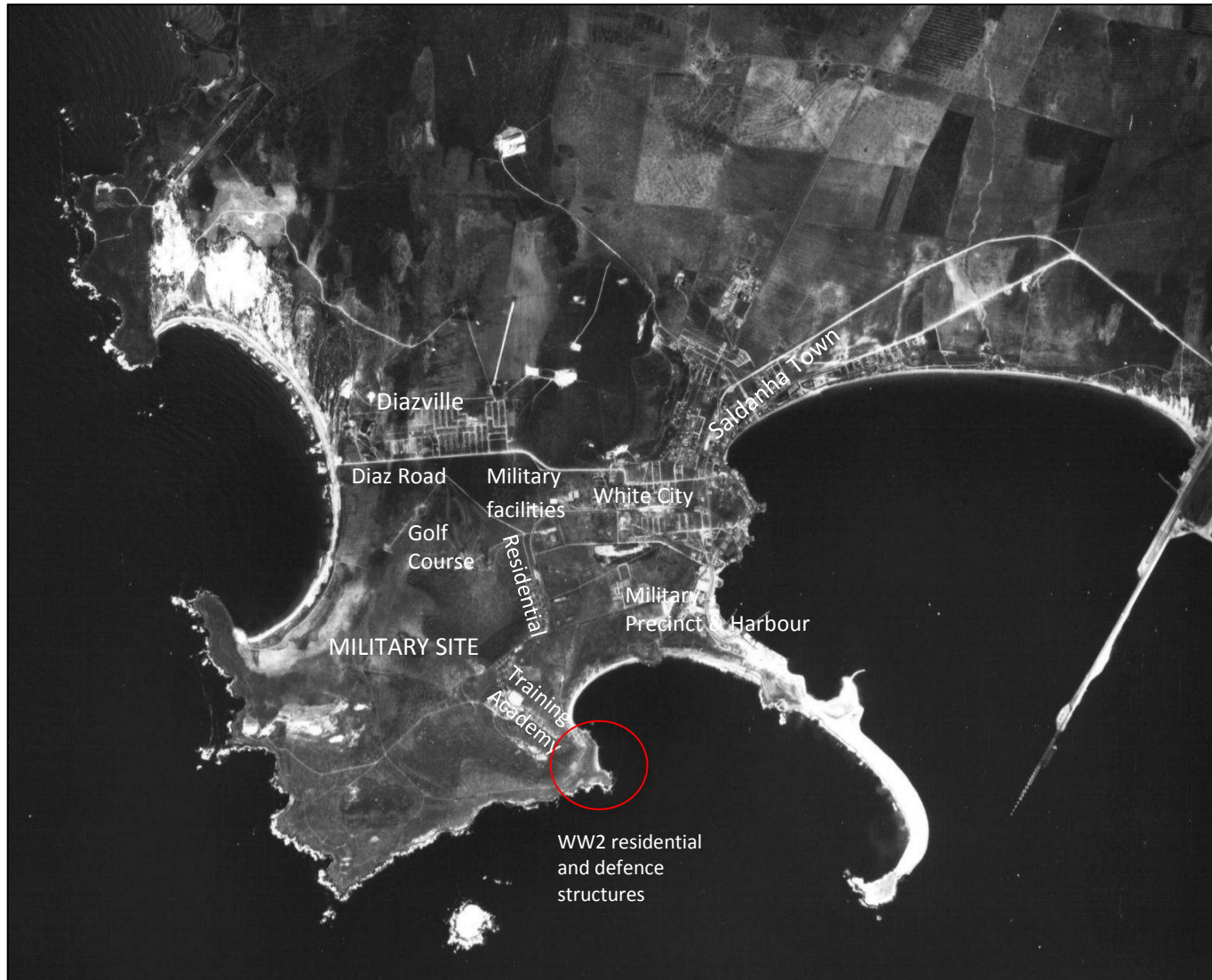
Aerial Photograph 2.4: 1980 image of Saldanha with Military Base visible with the increased in the development of Saldanha town, Diazville and White City Township with Diaz Road on the northern boundaries of the Military Base, National Geo- Spatial Information, Rural Development Department, 2013
