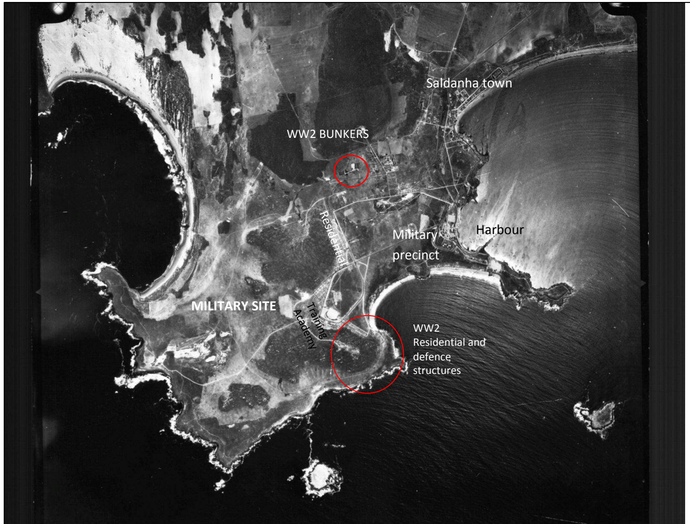
Aerial Photograph 2.2: 1960 image of Saldanha with Military Base visible with little development on its boundaries, National Geo- Spatial Information, Rural Development Department, 2013
