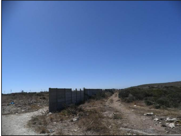
Photograph 4: Existing vibracrete wall that defines the site and municipal land.
