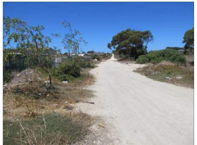
Figure 18. View facing east.
