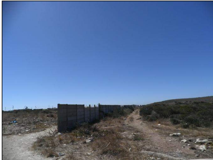
Photograph 2.9: Saldanha Military site: existing vibracrete wall defining site and municipal land, position of proposed wall, 2013 O'Donoghue
