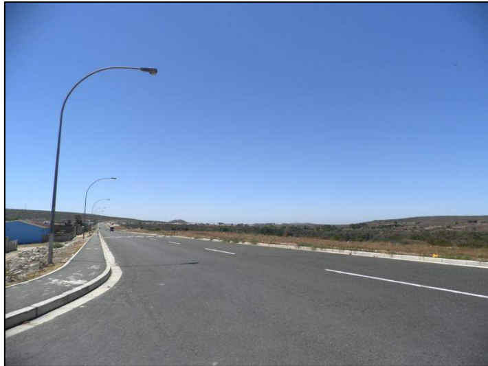
Photograph 2.12: Saldanha Military site: Diaz Road with site (right) and residential suburb Diazville (left). Proposed wall will be constructed on site boundary where existing damaged fence is located, 2013 O'Donoghue
