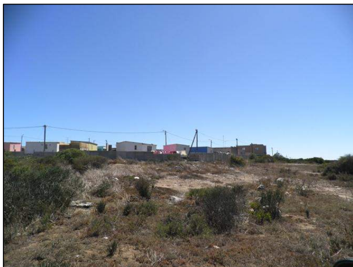
Photograph 2.11: Saldanha Military site: existing vibracrete wall defining site and formal housing development, position of proposed wall on boundary of urban development, 2013 O'Donoghue
