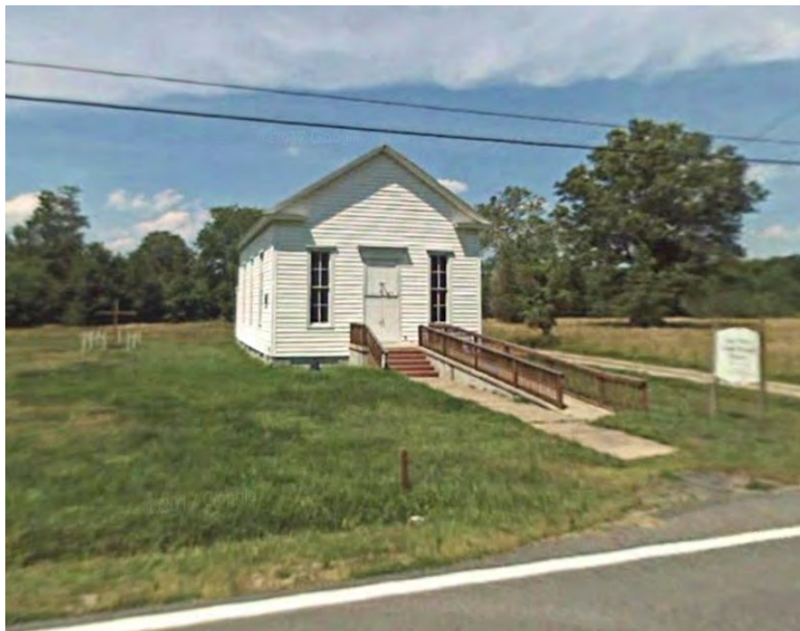
John Wesley Methodist Church Located on Capitola Road in Tyaskin. This church is at-risk to the 1% annual chance flood event.
