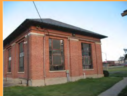
Photograph 2-1: Pump Building Looking from the East
