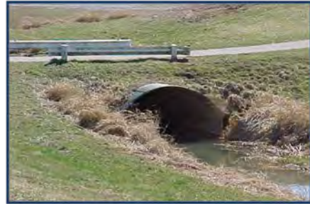
Before Mitigation and After Mitigation
