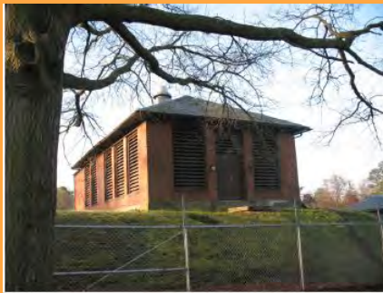
Photograph 2-3: Aerator Building Looking from the North
