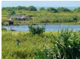
Natural vegetation is cleared to start construction
