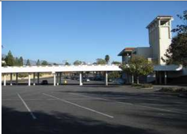
Approximately 16 acres of surface parking lots surrounding La Cumbre Plaza is an area of substantial potential future growth.
