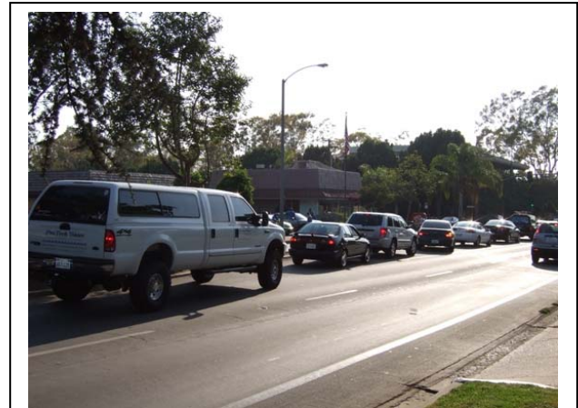
Peak-hour traffic on upper State Street can exceed the capacity of left turn pockets and obstruct through traffic.
