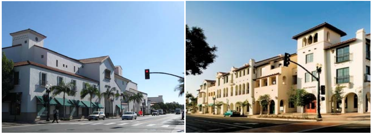
Construction of new development such as the 1990s-era Paseo Nuevo and Paseo Chapala, constructed in 2005, have the potential to result in substantial changes in the character of El Pueblo Viejo, including less openness, loss of mountain views, and a change in the City's small-town character. Plan Santa Barbara policies address building height, size, bulk, scale, and design, and would promote consistency with the current character of the Downtown.
