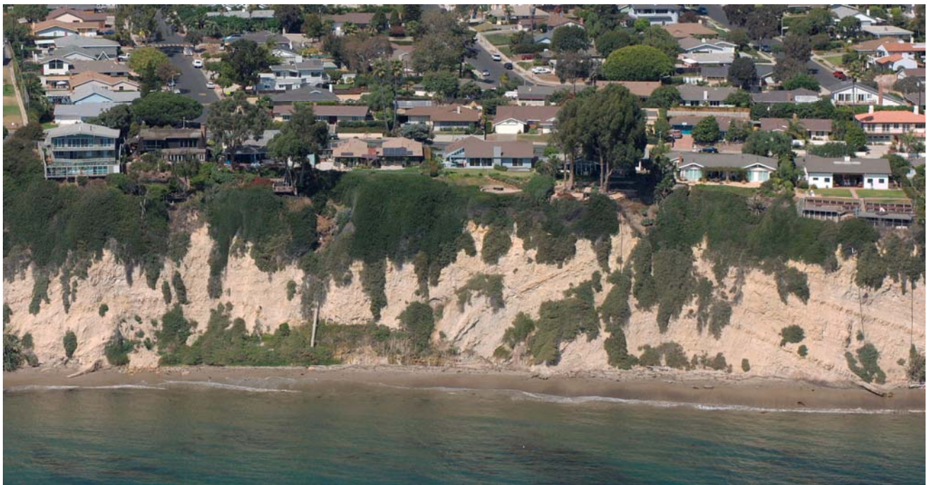
Approximately 75 existing homes in the City are located within the bluff retreat hazards zone, a number of which could be exposed to serious damage or destruction from sea cliff retreat over the next two decades. Many Mesa area homes have limited setbacks from the bluff edge. Climate change-induced sea level rise is projected to accelerate sea cliff retreat, which could expose more homes to damage by 2050, as well as portions of Shoreline Park and several public roads such as segments of Cliff Drive.
