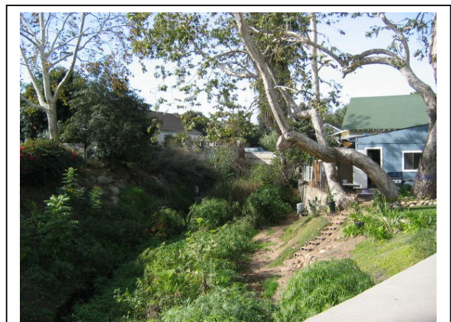
Mission Creek flows through central Santa Barbara and the close proximity of development can contribute to potential flooding and surface water quality problems.
