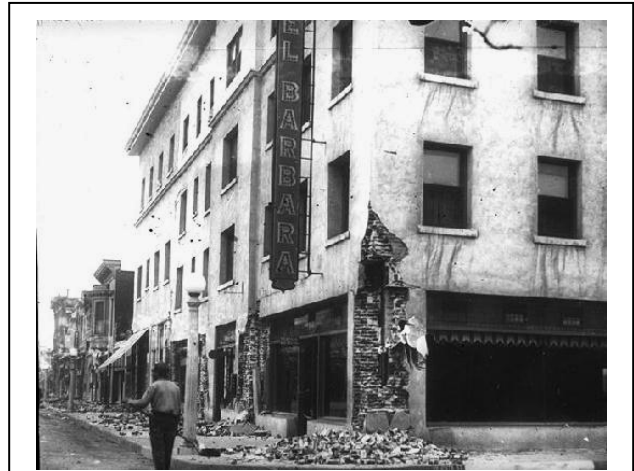
The 1925 earthquake caused significant damage to the City, including much of the Downtown and State Street (Earthquake Engineering Research Center).
