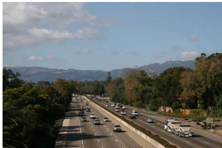
Traffic along U.S. Hwy 101 is a major source of noise within the City and is of particular concern where it borders residential neighborhoods such as near the Micheltorena Street overpass.
