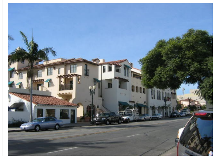
Historic Resources and Community Design policies would include new size, bulk, and compatibility standards to address urban design issues and community character, particularly those associated with new multi-story development.
