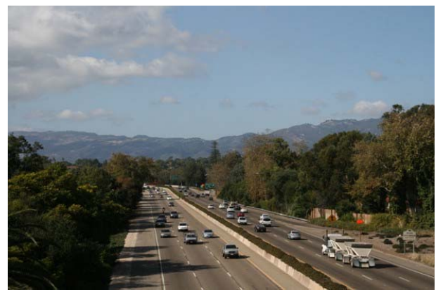
Traffic along U.S. Highway 101 is a major source of noise within the City and is of particular concern where it borders residential neighborhoods such as near the Micheltorena Street overpass.
