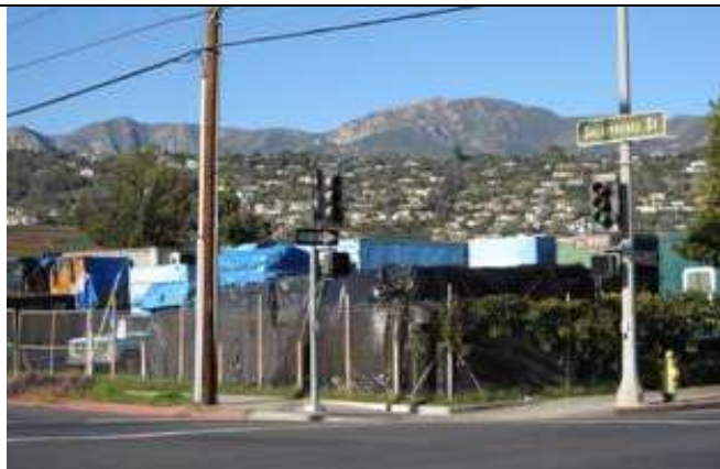
The 4.4-acre 600 block of East Haley Street supports service commercial businesses (e.g., Catholic Charities Thrift Store). However, based on the less developed nature of most of the site (e.g., low use truck yard), this block is a potential area of future growth.
