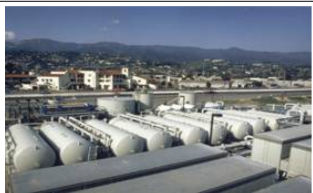
The City's Desalination Facility is currently in long-term storage, but could be reactivated to produce 3,125 AFY of water during a critical drought.
