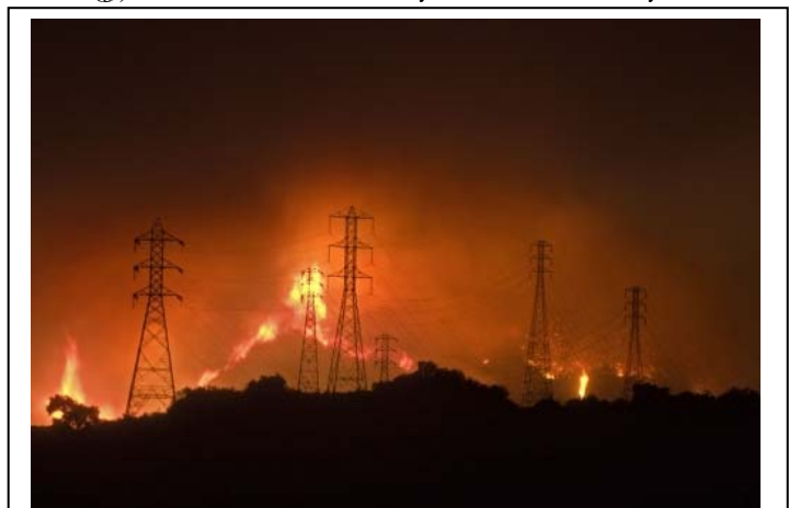
The City can experience power outages from wildland fires adjacent to foothill 66 kV transmission lines (2008 Tea Fire; The Independent 2008).
