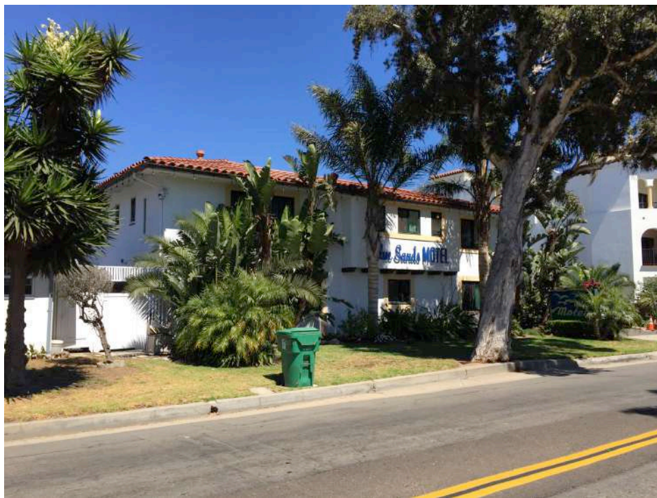
LOOKING TOWARDS NORTHWEST ELEVATION OF STRUCTURE
