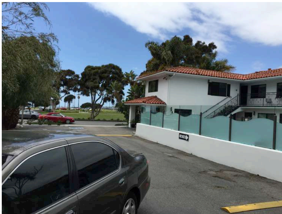
LOOKING WEST TOWARDS (E) STRUCTURE AND (E) POOL FROM PARKING LOT
