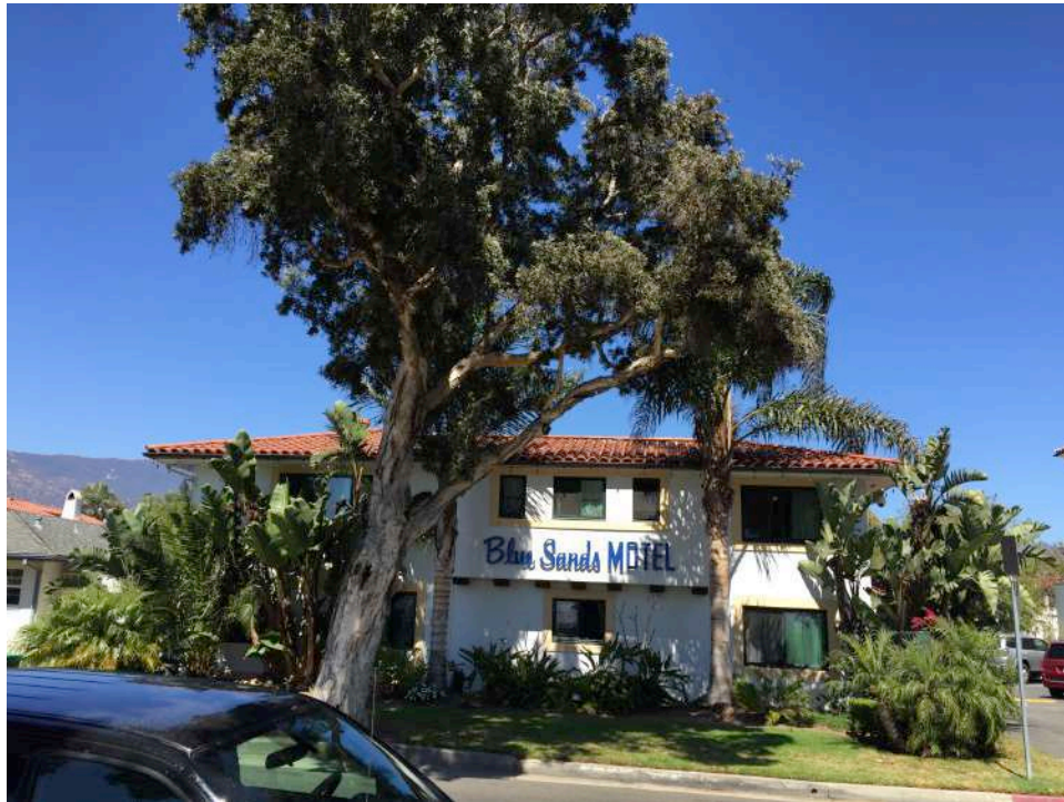
LOOKING EAST TOWARD WEST ELEVATION OF STRUCTURE
