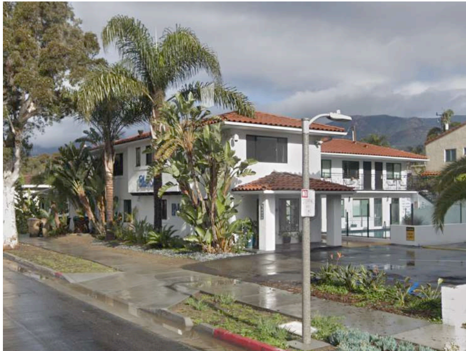
LOOKING TOWARDS SOUTHWEST ELEVATION OF STRUCTURE
