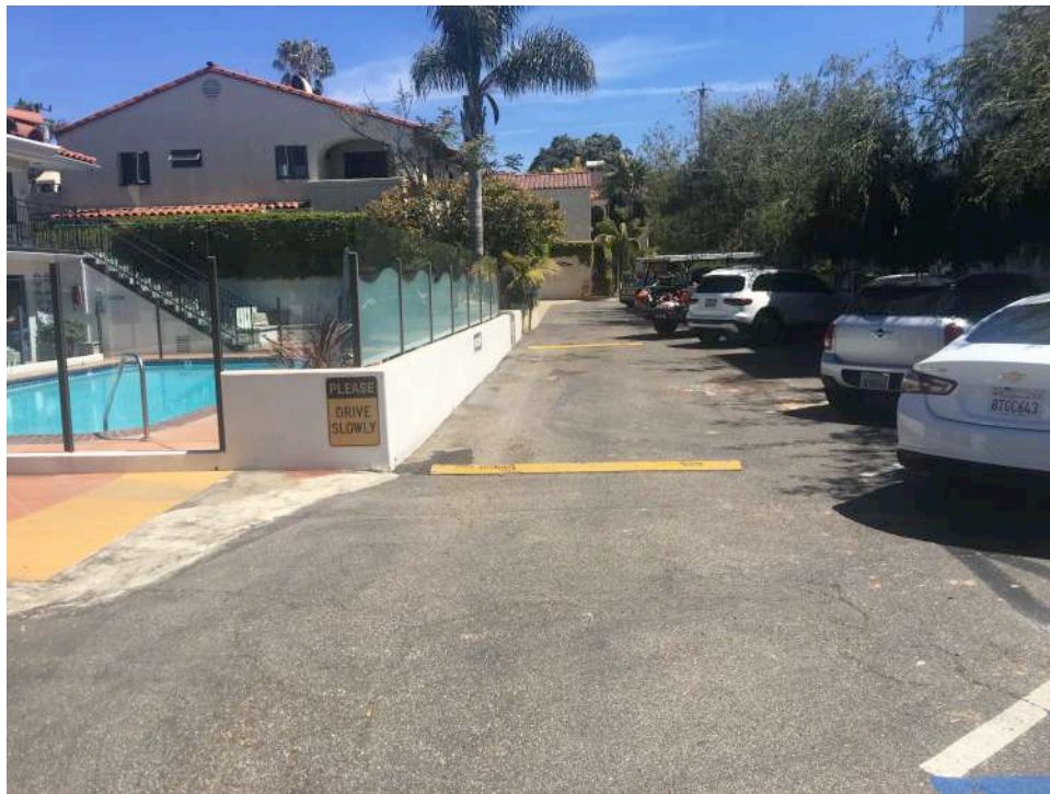
LOOKING NORTHEAST TOWARDS (E) PARKING LOT FROM DRIVEWAY
