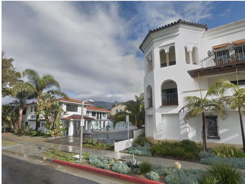
ADJACENT STRUCTURE AT SOUTH OF PROPERTY
