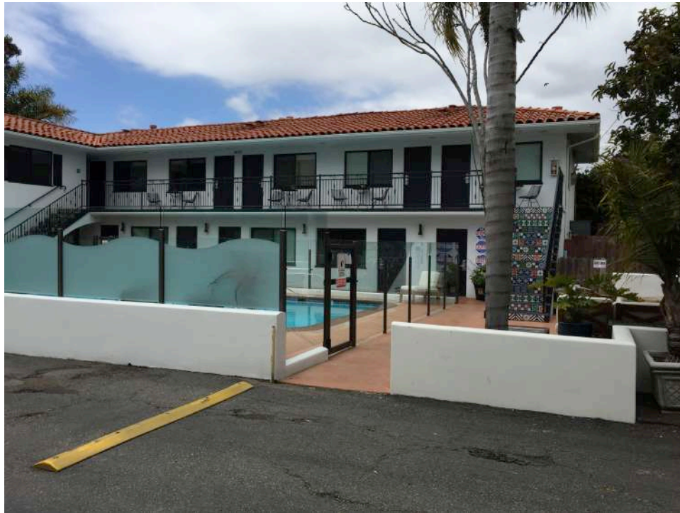
LOOKING TOWARDS SOUTH ELEVATION OF STRUCTURE FROM PARKING LOT
