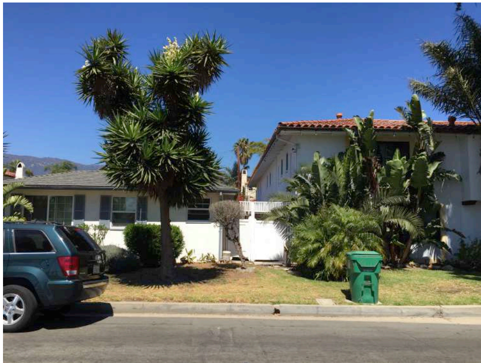
ADJACENT STRUCTURE AT NORTH OF PROPERTY
