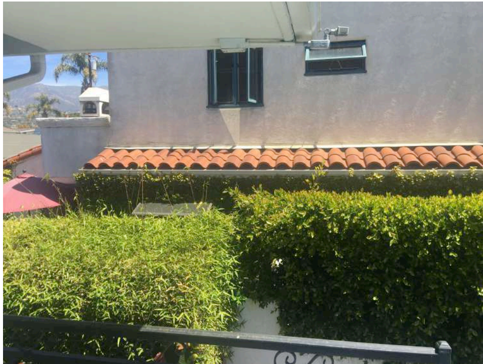
LOOKING NORTHEAST TOWARD ADJACENT STRUCTURE FROM EAST STAIR TOP LANDING
