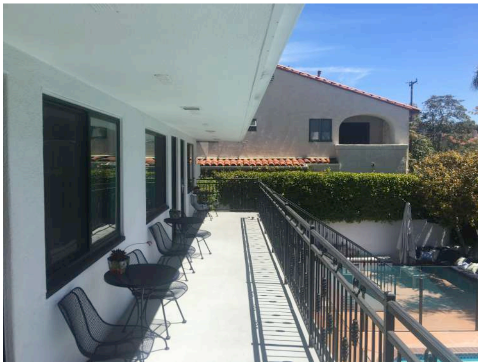
LOOKING NORTHEAST TOWARD ADJACENT STRUCTURE FROM WEST STAIR TOP LANDING
