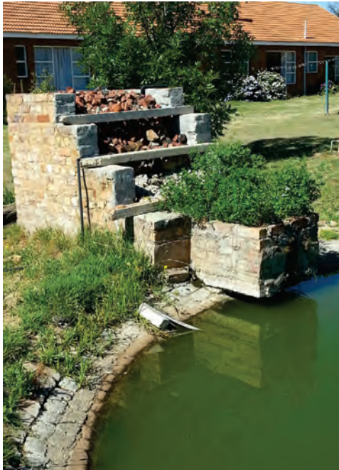
Home-made domestic grey-water filter. Note algae-laden green water in pond.
