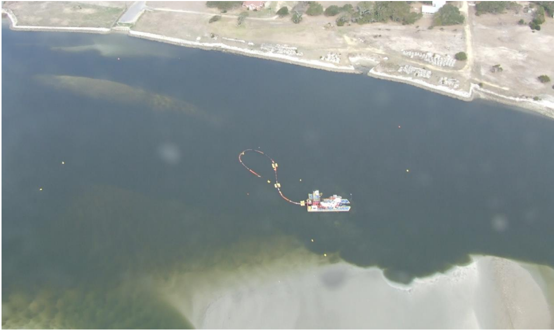
Photo 2.3. 2014 USACE LFIX maintenance dredging.
