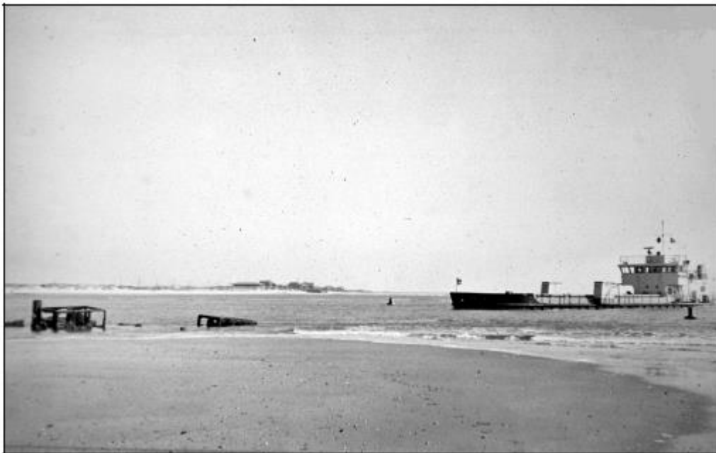
Photo 4.4. Exposed boilers of the Bendigo (left foreground) and the USACE dredge boat, Currituck, Site 0001LFI.
