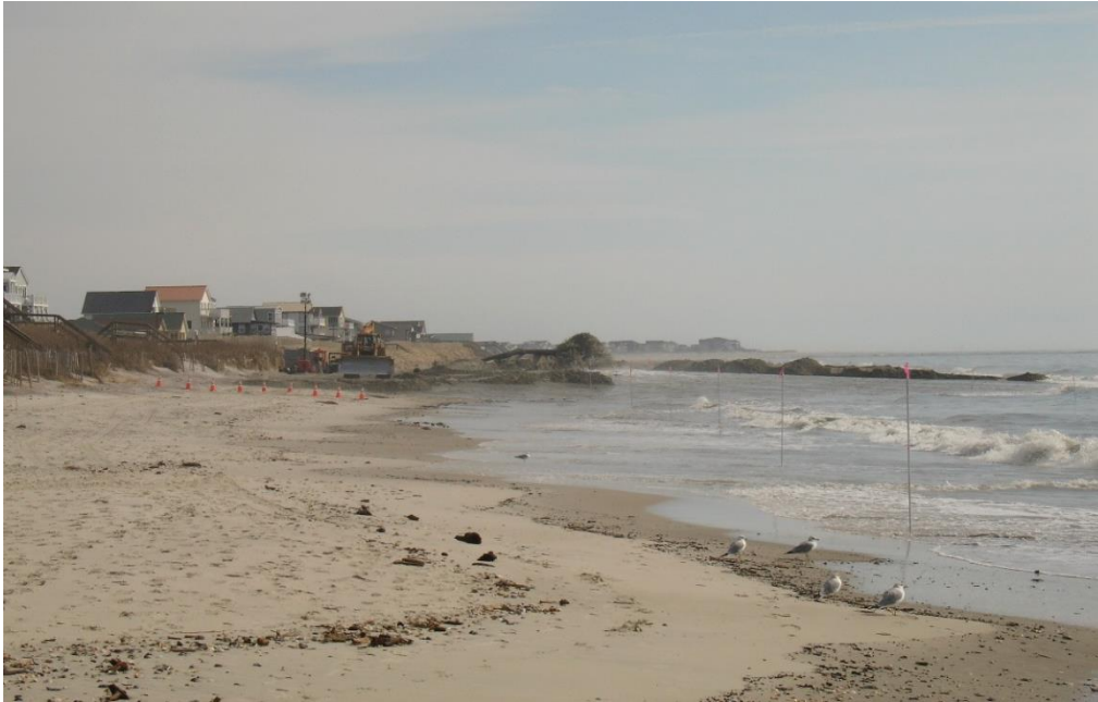
Photo 3.1. View of temporary containment berm during the 2014 beneficial use project on the East End.
