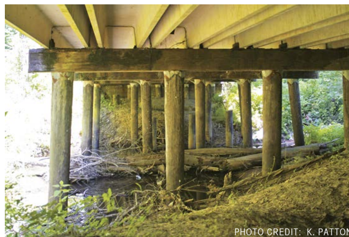
Figure 16. A bridge with a construction design suitable for roosting bats.
