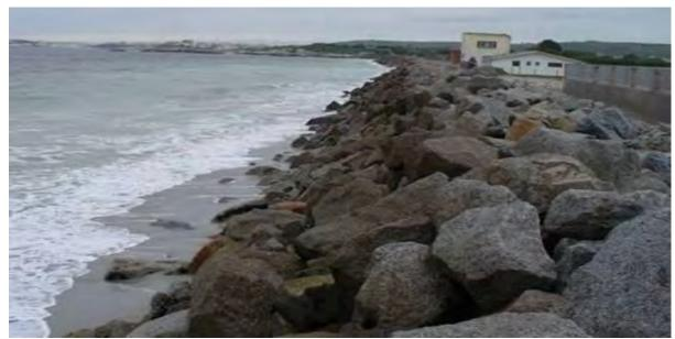
Figure 5.7. Rock revetments constructed along the beach at Langebaan in an effort to protect coastal infrastructure.
