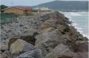
Figure 5.1. A) Under natural circumstances, dune vegetation can "move" with the beach as it erodes and accrete under the influence of natural processes. B) Protection of infrastructure erected too close to the high water mark, on the other hand, necessitates construction of artificial barriers and leads to the loss of the beach ecosystem and associated amenities.
