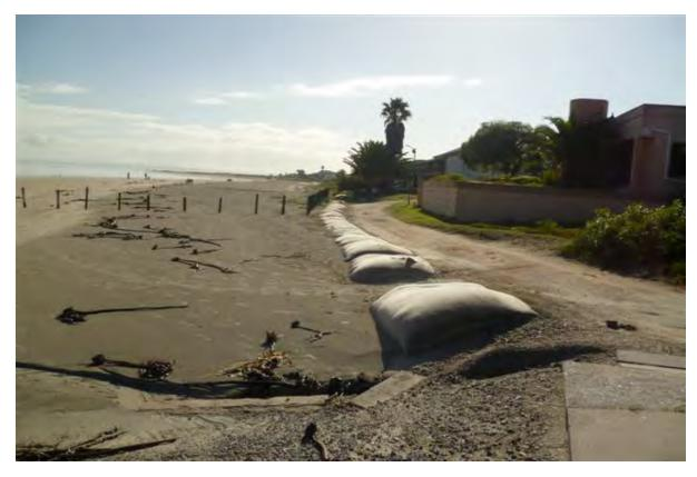
Figure 5.10. Erosion protection measures at the Alabama Street Slipway. Source: Common Ground Consulting (2013).
