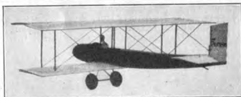
Farman „Sport“ (1922) E: H. Farman, Billancourt; A: Farman Frères, Billancourt. S: 1; St: Schw.; Bst: H. — l = 7,00 m; b = 9,00 m; F = 25,00 m 2 ; Gr = 125,00 kg; Gz = 70,00 kg; G = 195,00 kg; G/F = 7,80 kg/m 2 .
