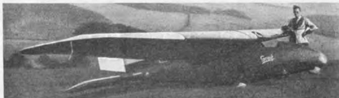
Hannover „Greif“ (1922) E: W. Blume, F. Hentzen, A. Martens, Hannover; A: Hannoversche Waggonfabrik, A.-G., Hannover. S: 1; St: Schw.; Bst: H; P: Göttingen; vg = 13,00 m/s; Gwkl = 1:18 ; vs = 0,72 m/s. — B.-L.: D: 0:45:0 h. — l = 5,52 m; h = 1,20 m; b = 11,60 m; t = 1,80 m; b/t = 1:6,3 ; F = 16,00 m 2 ; Hr = 1,80 m 2 ; Sr = 0,60 m 2 ; Tg = 34,00 kg; Lg = 6,40 kg; Rg = 46,00 kg; Fg = 6,40 kg; Gr = 92,80 kg; Hg = 70,00 kg; G = 162,80 kg; G/F = 10,60 kg/m 2 .
