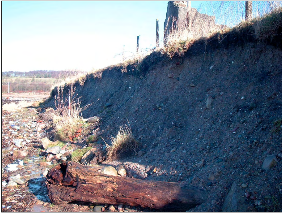
Plate 15- Eroding cliff east of Craighendoran. (Unit 2, Erosion Class, Clyde Map 1)
