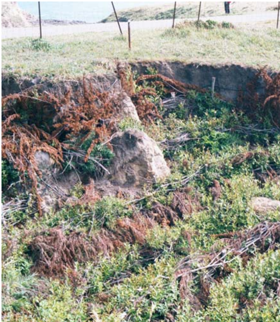
Photo 3 – Willow wattles at Smithy slump
