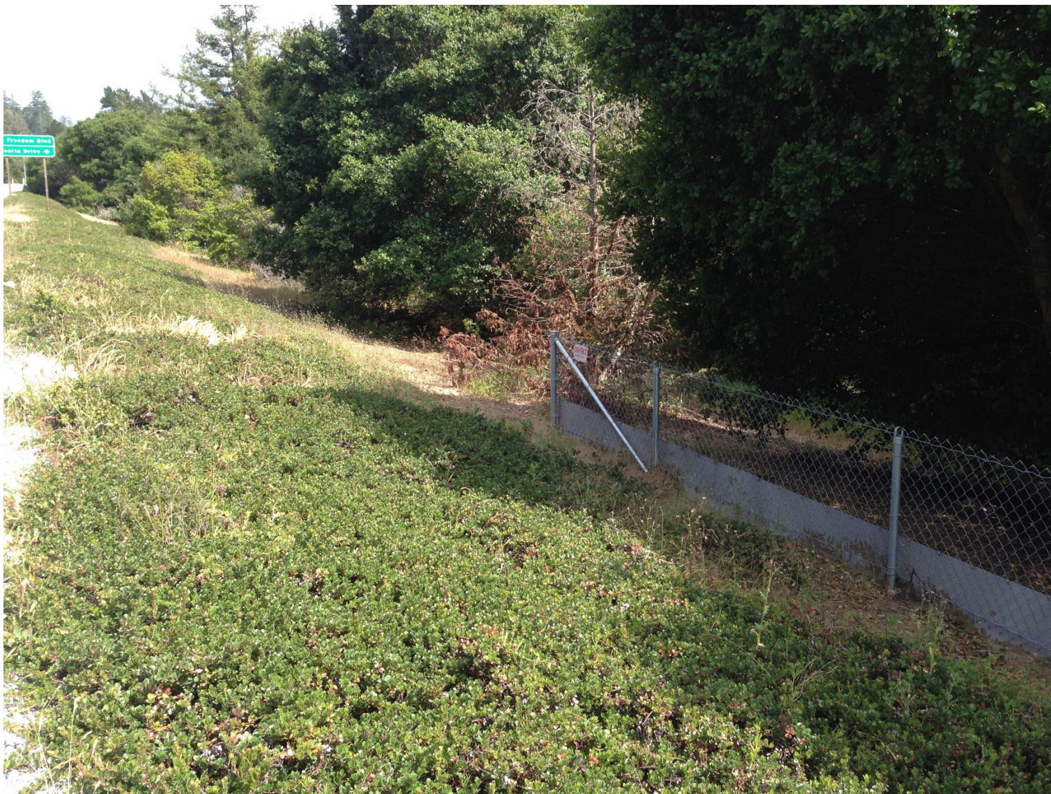
Figure 6. Photo showing the southern end of the exclusion fence near Freedom Boulevard. Note the open access to the shoulder.
