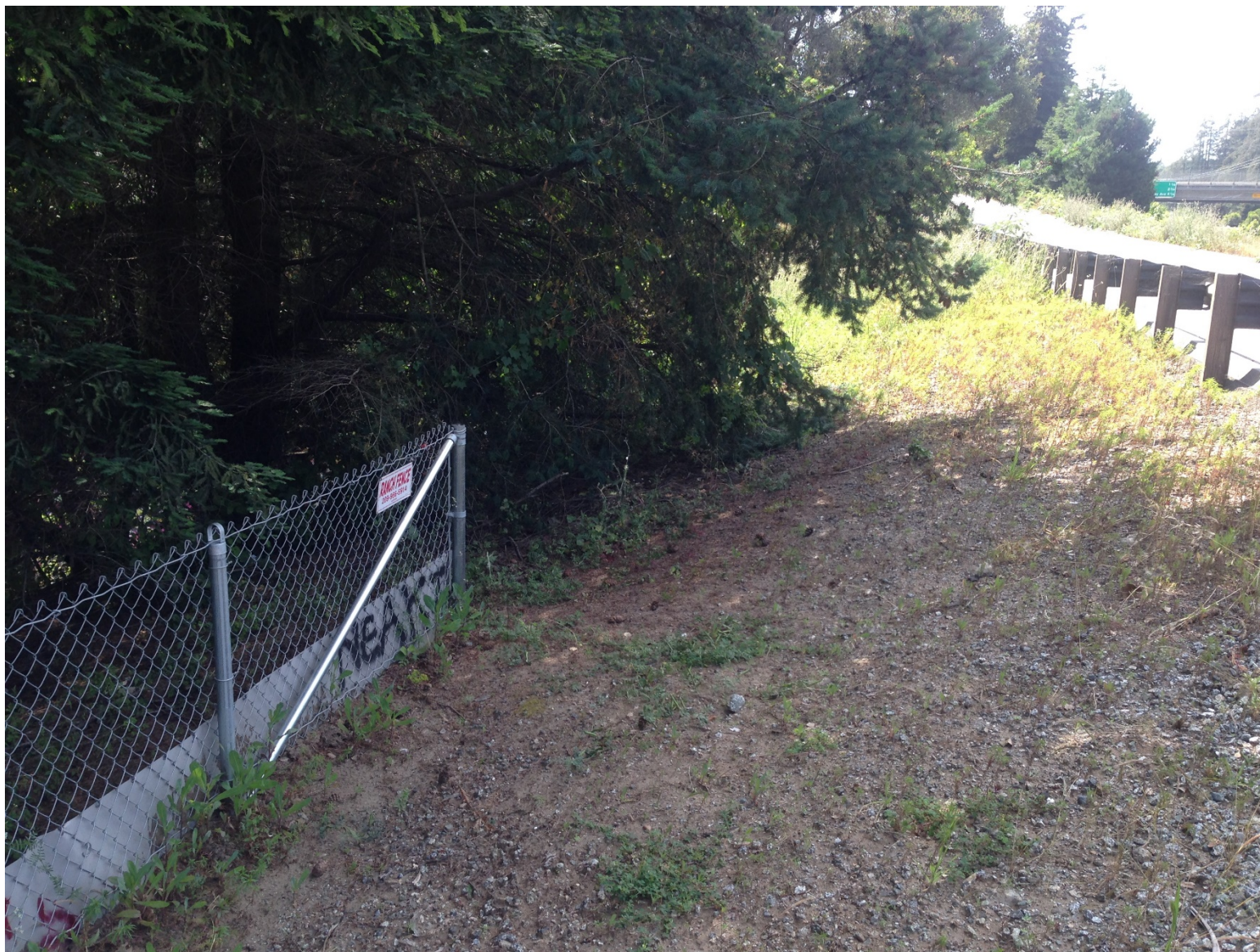
Figure 5. Photo showing the northern end of the exclusion fence near Rio Del Mar Boulevard. Note the open access to the shoulder.
