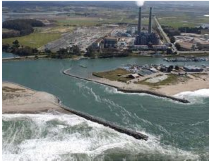
Figure 2. Moss Landing Harbor levees
