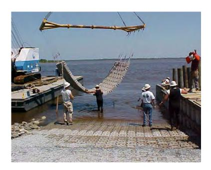
PHOTOGRAPH 4-1 INSTALLATION OF ACBS BY CRANE
