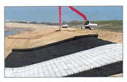
The upstream strips of material must overlap the downstream strips and upslope strips overlap down-slope strips. (See Diagram 4)
