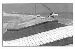
The upstream strips of material must overlap the downstream strips and upslope strips overlap down-slope strips. (See Diagram 4)
