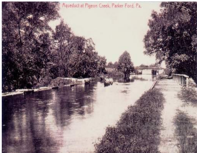
Undated photo of the Aqueduct at Pigeon Creek. Looking north.
