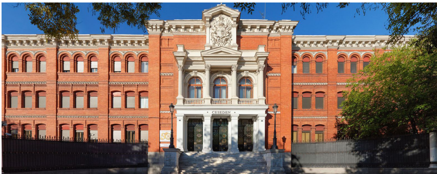
Figura 6. Fachada principal del Centro Superior de Estudios de la Defensa Nacional Front of the building of the Centre for Higher National Defence
