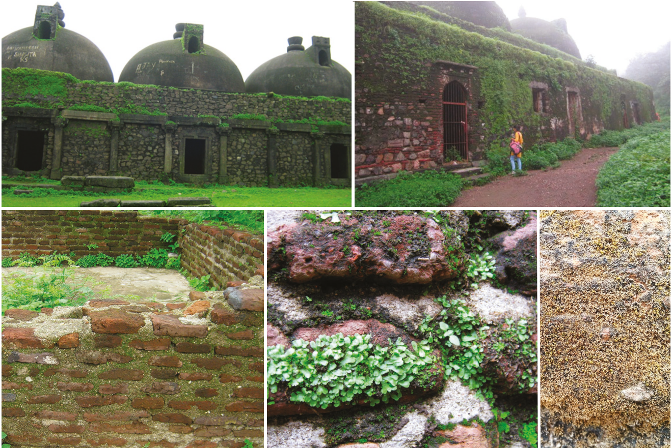
FIG. 1. — Glimpses of sites showing biological colonization and deterioration of the monuments of Champaner Pavagadh.
