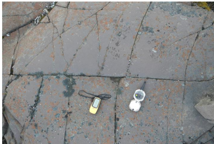
Fig. 3-5 Note how the rock is broken into rectangular blocks, a common phenomenon when two orthogonal (at right angles) joint sets exist. Also note how the one set of joints truncates against the continuous joint running from side to side in the image. If this relationship is consistent, the continuous joint is the longitudinal joint, which is interpreted to have formed before the cross joints that truncate against it. Finally note that some fractures that can not be assigned to one of the two orthogonal sets exist. It is not uncommon at all that a rock body can have three or more joint sets developed within it.
