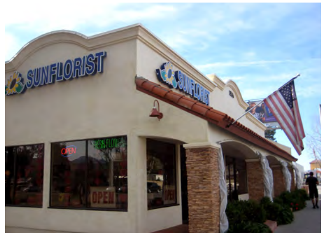
Example of shopfront frontage at Soledad Canyon Road and Solamint Road
