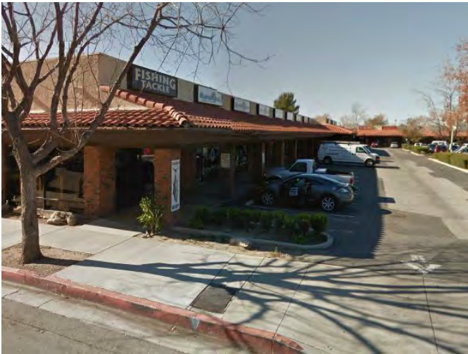
Examples of gallery frontage on Soledad Canyon Road
