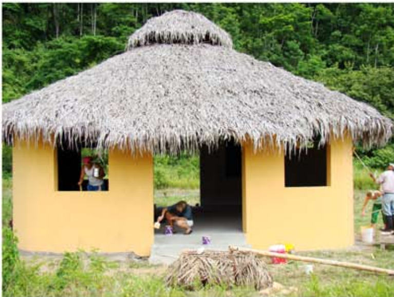
EcoCenter construction - April 2008 (view to the East)
