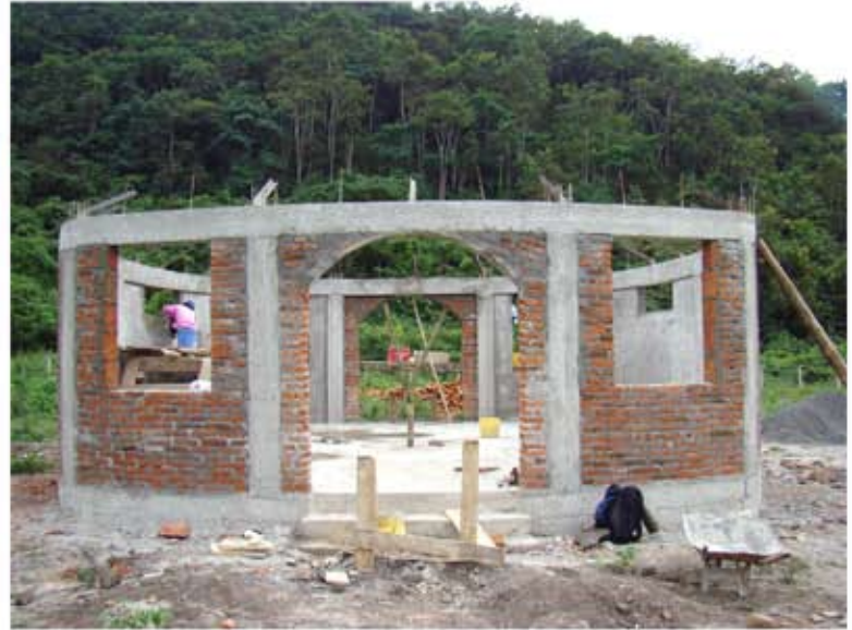
EcoCenter construction - July 2007 (view to the West)
