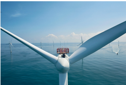
Horns rev 3 in Denmark, built and owned by Vattenfall. The park holds 49 plants and has a capacity of 406 MW, which means the approximate annual consumption for 425,000 Danish households. Source: Vattenfall, 2018.
