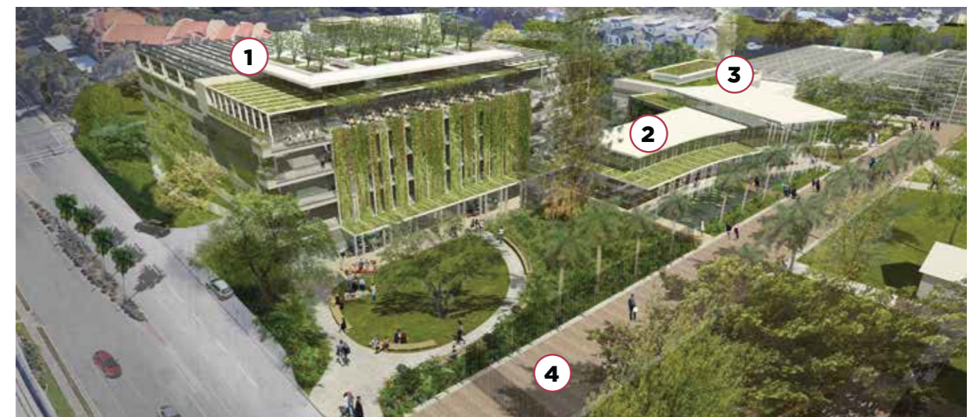
The first phase of the three-phase master site plan includes the Sky Garden and Parking Terrace (1), which includes our plant shop, (2) Jean Goldstein Welcome Center and Nathalie McCulloch Research Library; and the Steinwachs Family Plant Research Center (3) for housing our preserved collections and administration offices. (4) Palm Avenue is preserved as a pedestrian-only thoroughfare through the Gardens.
