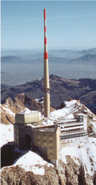
Sântis transmitter in Switzerland VHF and TV antenna systems completely enclosed in a heated GRP radome.
