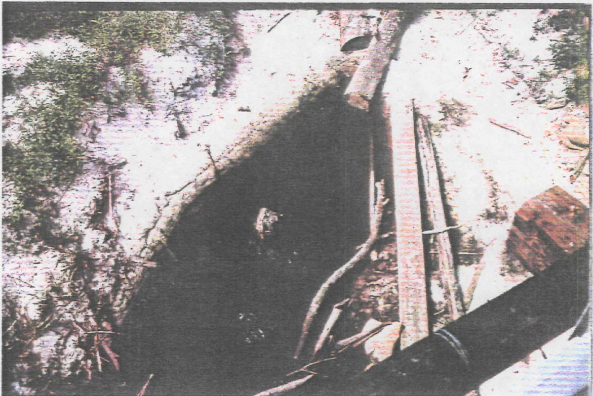
Exposure No. 6, Middle Zone of Cold Creek Swamp at Virginia Chemicals Road Bridge
