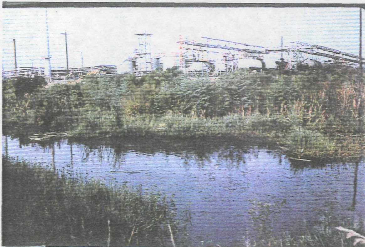
Exposure No. 4, Upper Zone of Cold Creek Swamp Showing Standing Water of Unnamed Tributary to Cold Creek. ICI Americas Cold Creek Chemical Plant is in Background
