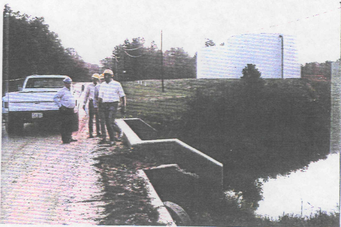
Exposure No. 2, Amoco Road Bridge -- Upper Swamp Zone
