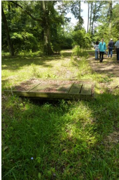
Photograph No. 30 Description: Southwestern portion of Combustion, Inc. site. Note wooden bridge over small ditch leading to the surface drainage. Date: May 20, 2010
