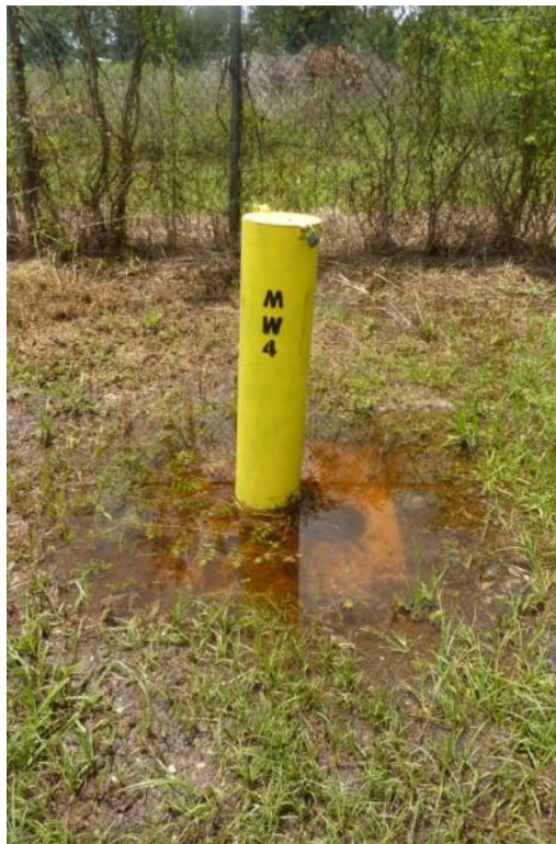
Photograph No. 40 Description: Monitoring well MW-4 in standing water. Date: May 20, 2010
