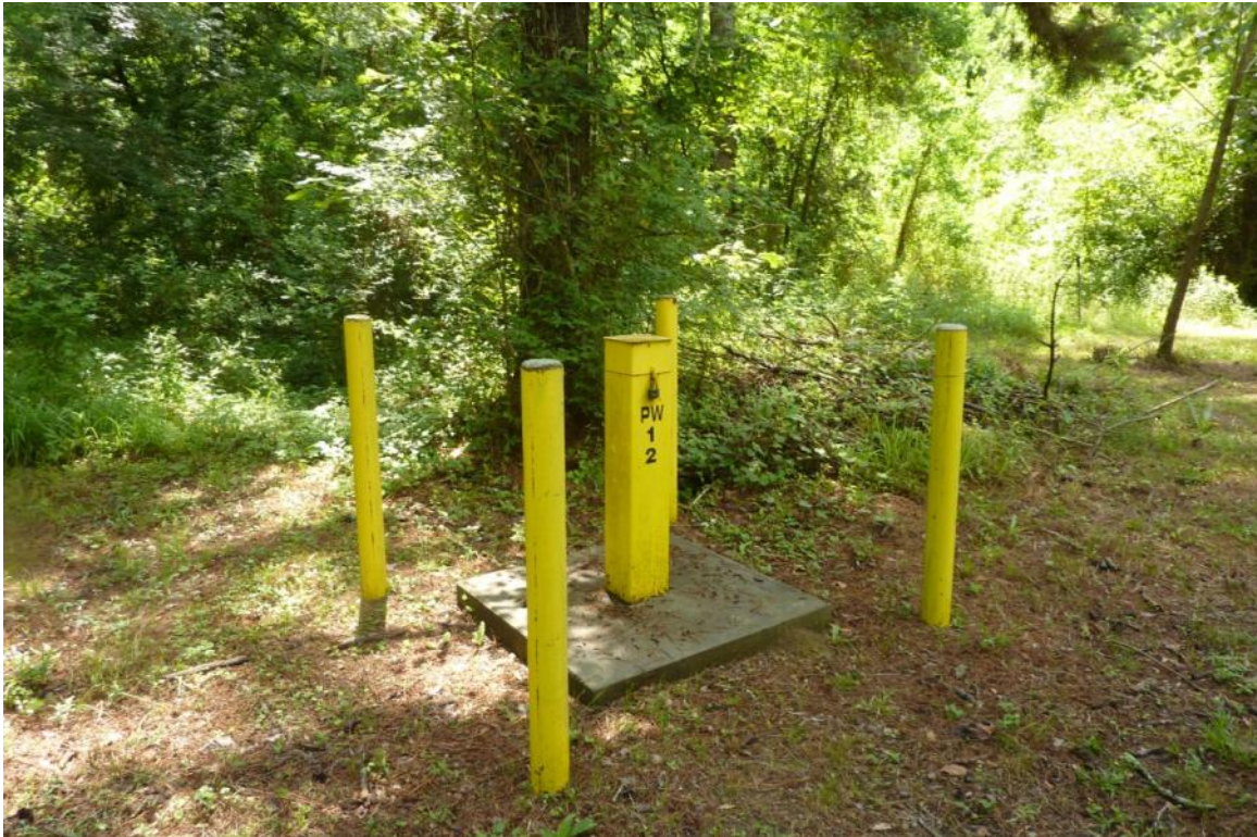
Photograph No. 29 Description: Piezometer PW-12. Date: May 20, 2010
