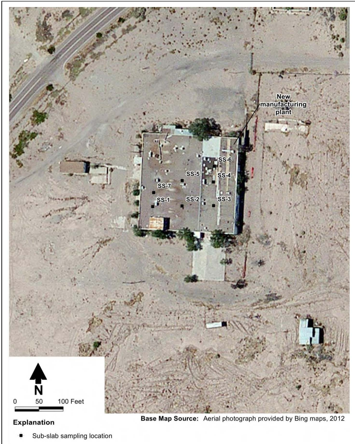
Figure 7. Sub-slab Sampling Locations
