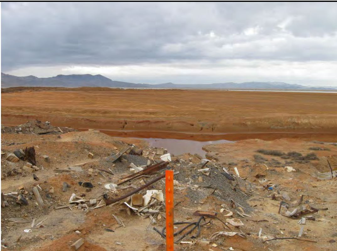
Photograph: 8 View of the former diversion ditch off the north flank of the landfill where it is connected to the main wastewater ditch (looking northwest). The t-post in the foreground shows alignment of transect B-B' with the former diversion ditch. Location: Former Diversion Ditch Date: 3/6/14 ERM US Magnesium Tooele County, Utah
