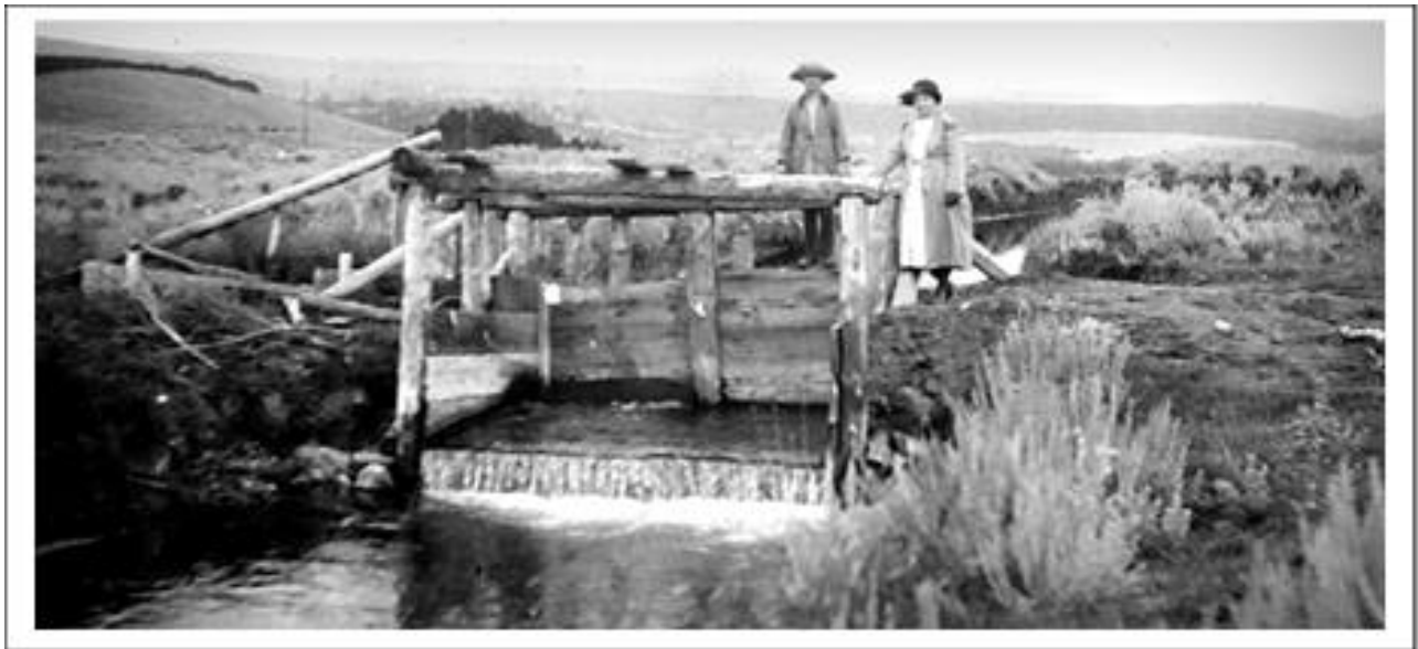
Figure 31: Irrigation Headgate near Brush Creek.
