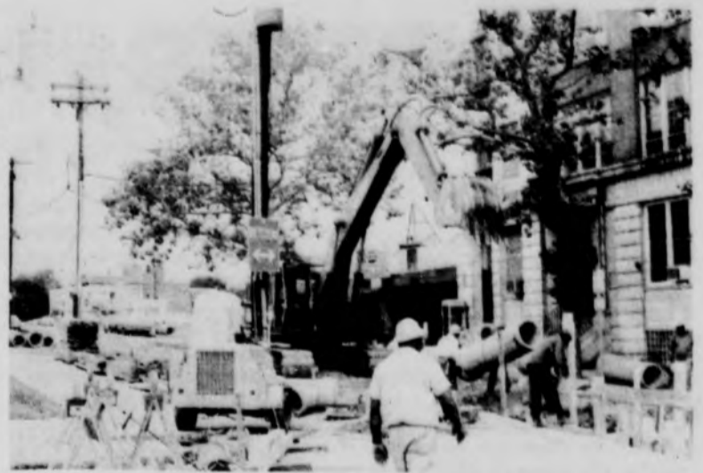
Work progressing on the sewer line in 32nd st.
