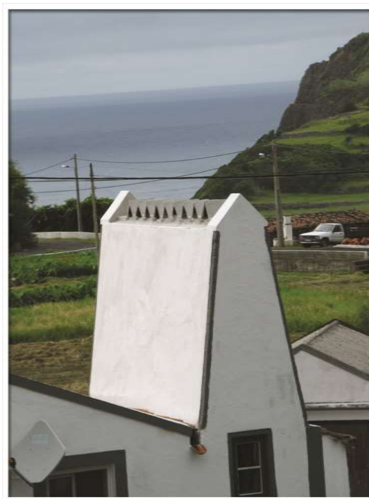
Figure 27. Details of a traditional chimney.
