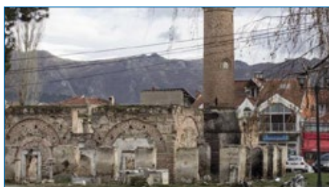
Figure 3: The burnt Carshi Mosque in Prilep. 23
